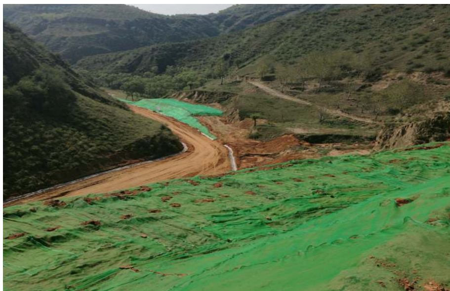
弃土场削坡分级及扰动面临时苫盖防护
